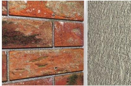
Wall to wall construction joint
